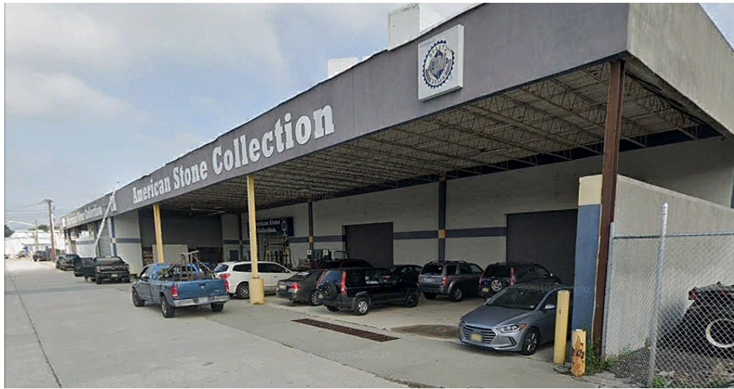
View of Front of the Property
