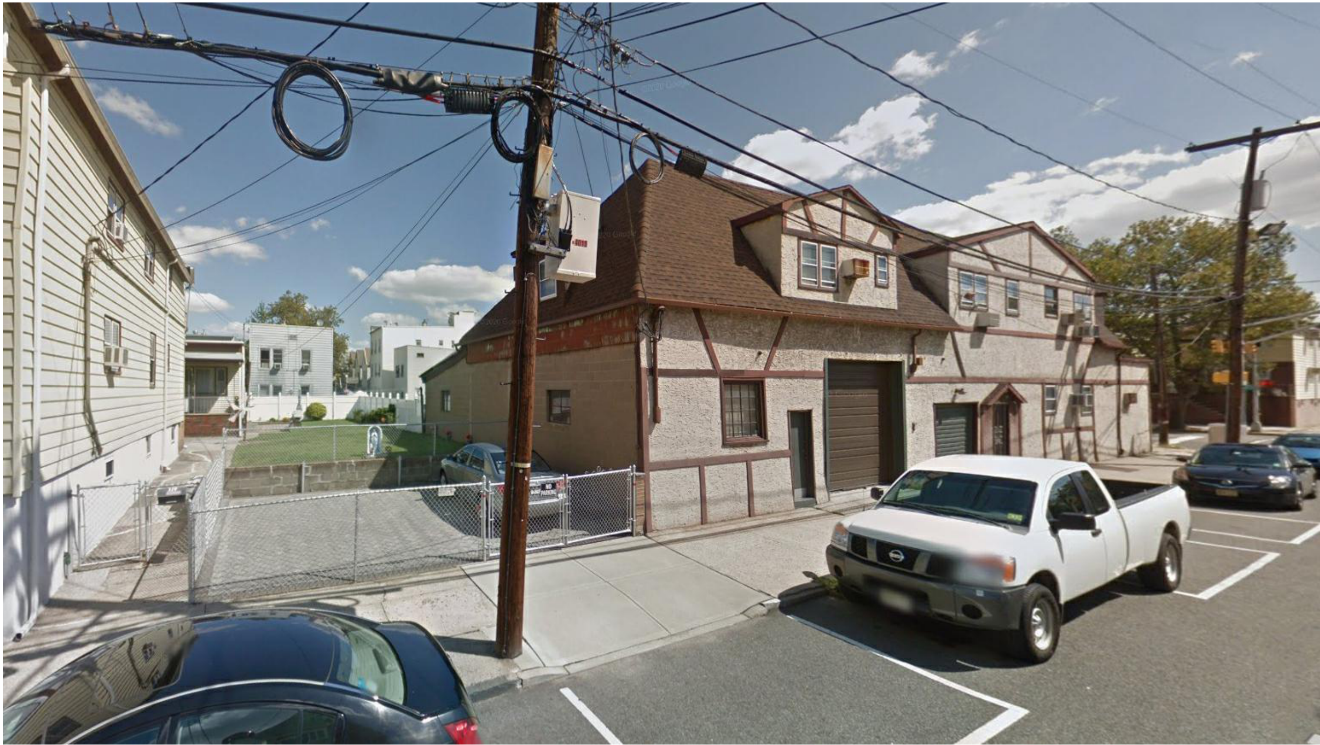
VIEW FROM W 12TH STREET
