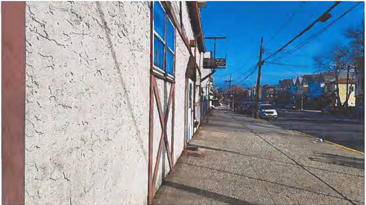
Figure 14 ~ View of blank walls along JFK Boulevard (taken on January 14, 2024)
