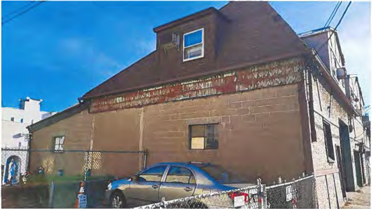
Figure 5 ~ View of west façade from 12 th Street frontage (taken on January 14, 2024)
