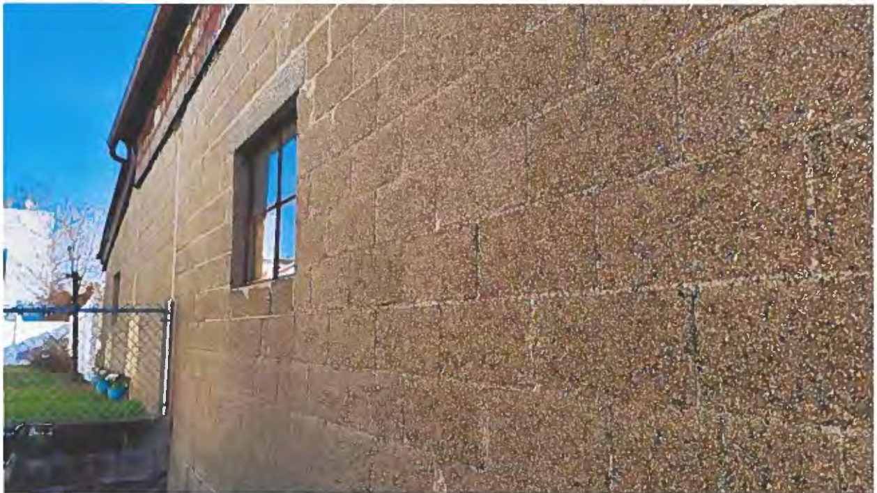
Figure 6 ~ View of west façade from 12 th Street frontage (taken on January 14, 2024)
