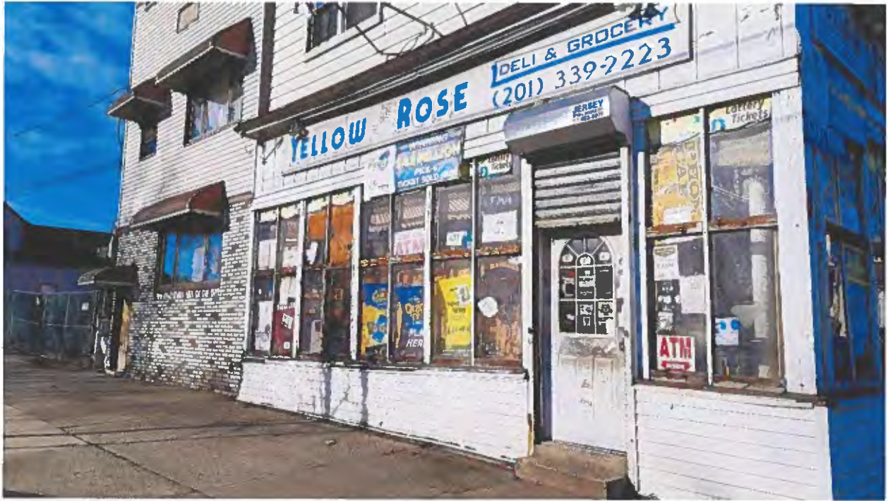
Figure 3 ~ View of subject building, on left, adjacent to the store in foreground (taken on January 14, 2024)
