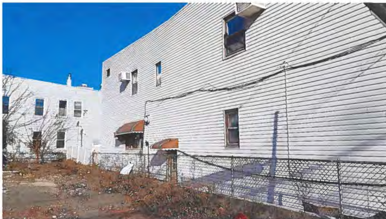
Figure 5 ~ View of south façade of subject building (taken on January 14, 2024)
