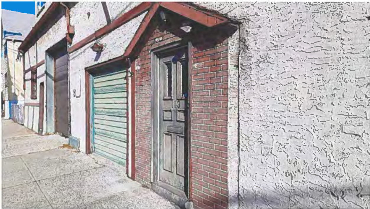
Figure 10 ~ View of multiple doorways and rollup loading door from 12 th Street frontage (taken on January 14, 2024)
