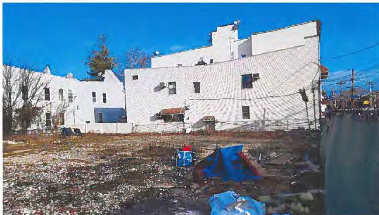
Figure 6 ~ View of south façade of subject building (taken on January 14, 2024)
