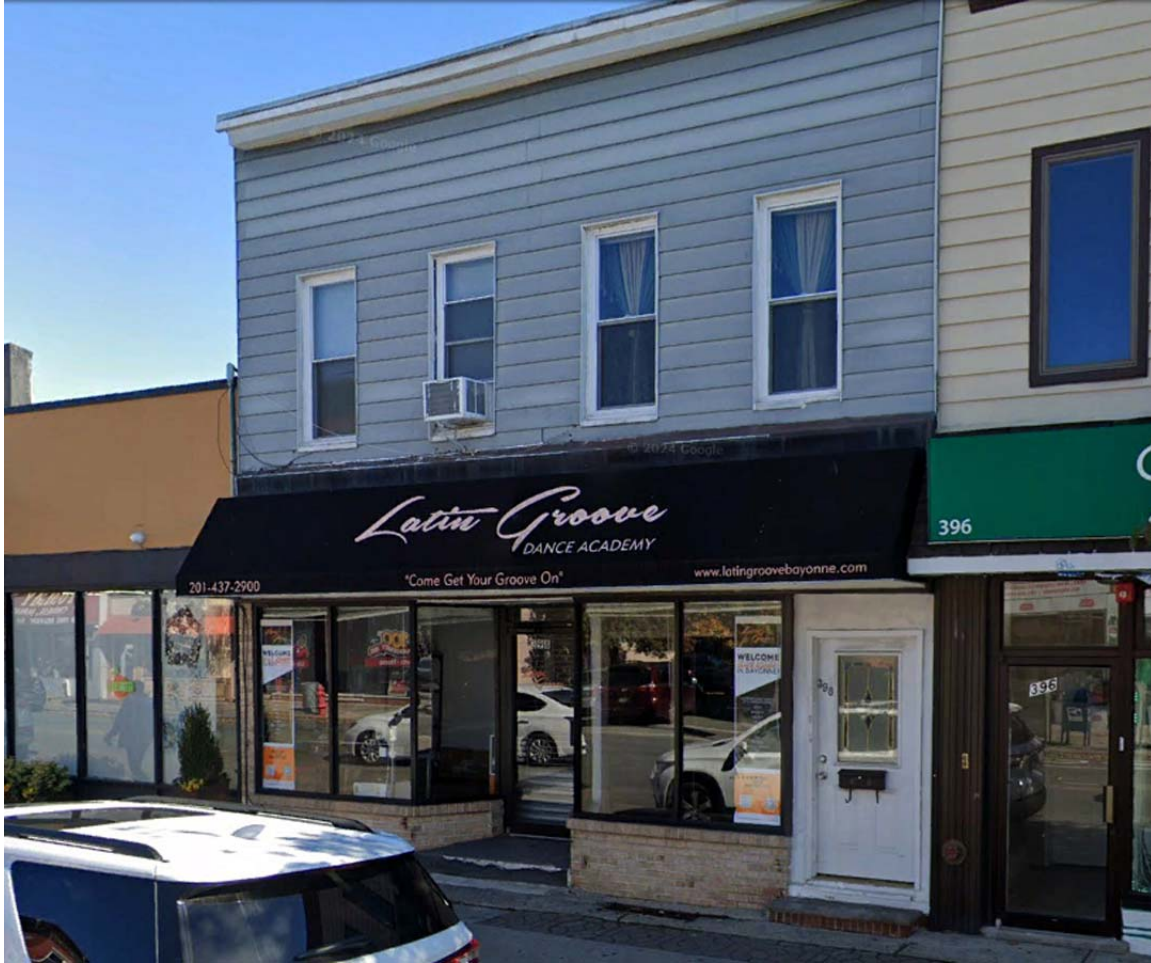
Front Façade of Building from Broadway
