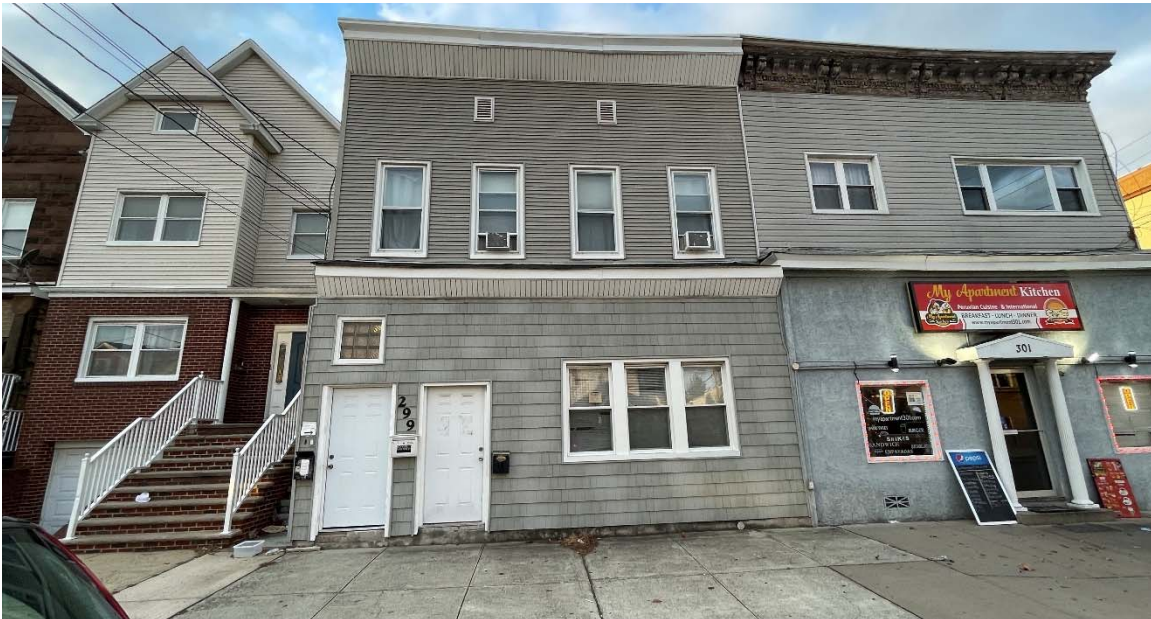
Fig. 1. Photo of Existing Building (Center) Front Façade
