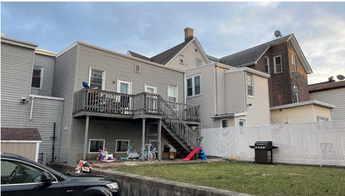
Fig. 3 View of Retaining Wall and Rear Yard of Subject Property
