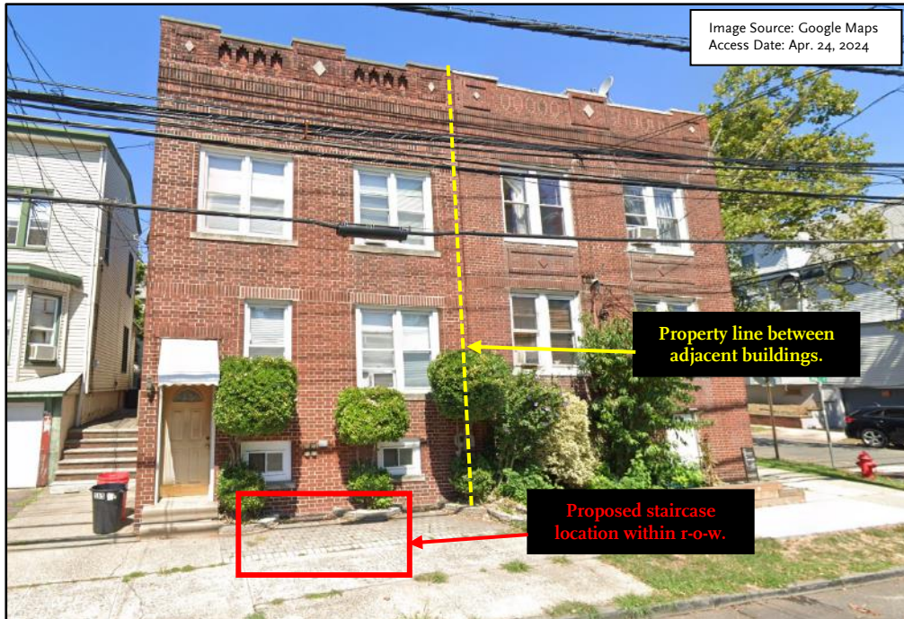
585 Avenue E Building Façade (PIQ)
