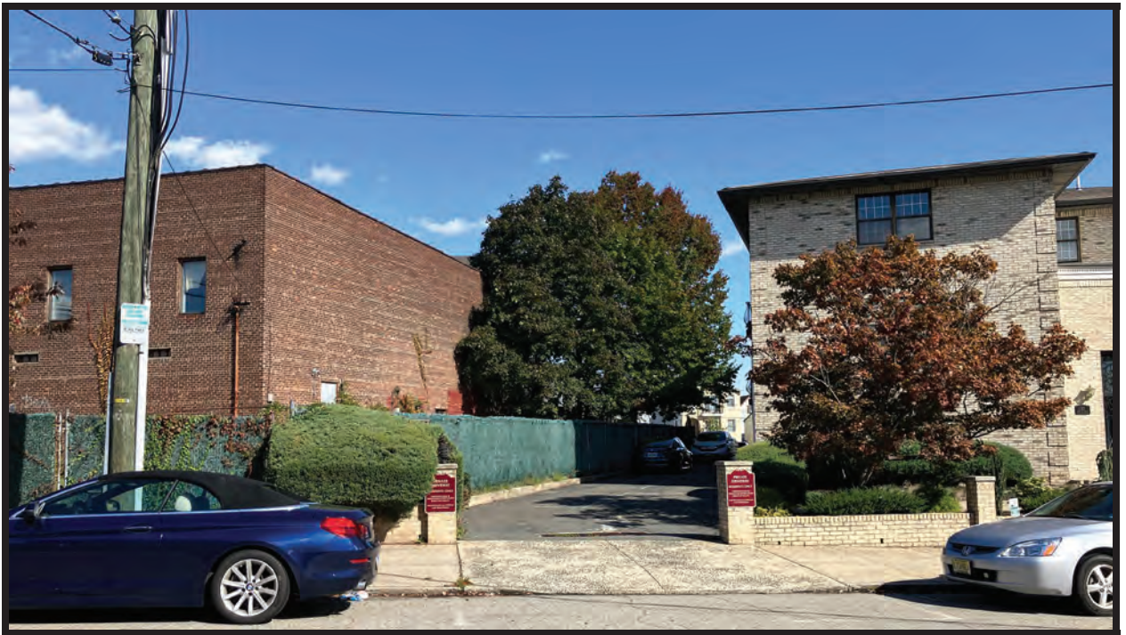
REAR OF PROJECT SITE VIEWED FROM WEST 48 TH STREET
