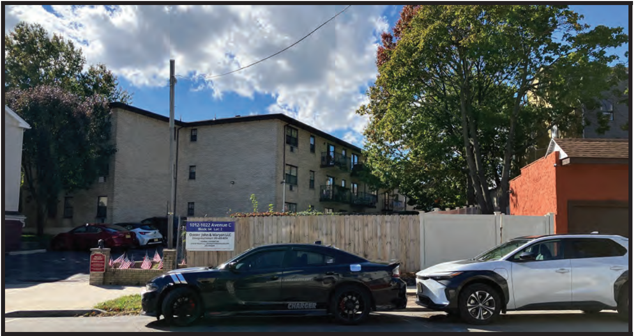
REAR OF PROJECT SITE VIEWED FROM WEST 49 TH STREET
