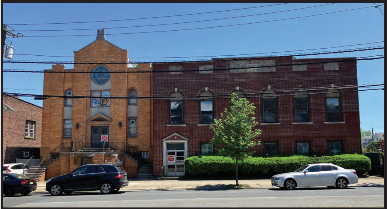
PROJECT SITE VIEWED FROM AVENUE C
