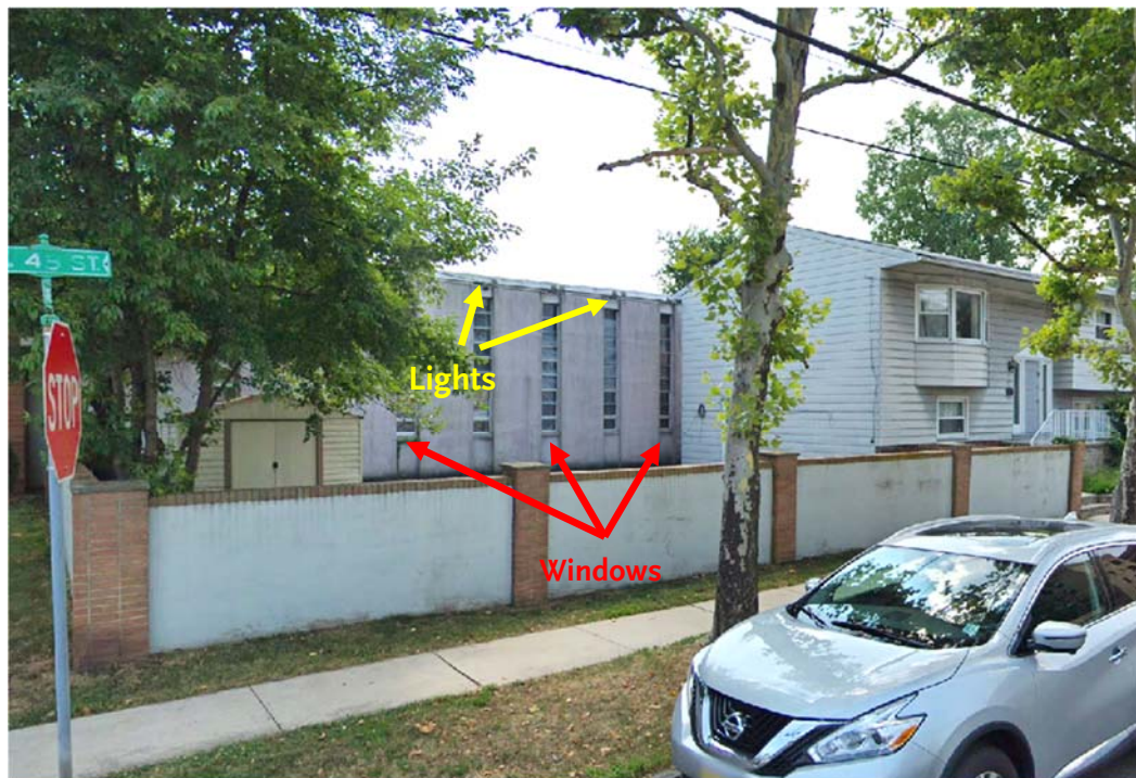
Lot 11.02 Looking Southwest from West 43rd Street (Source: Google Street View)
