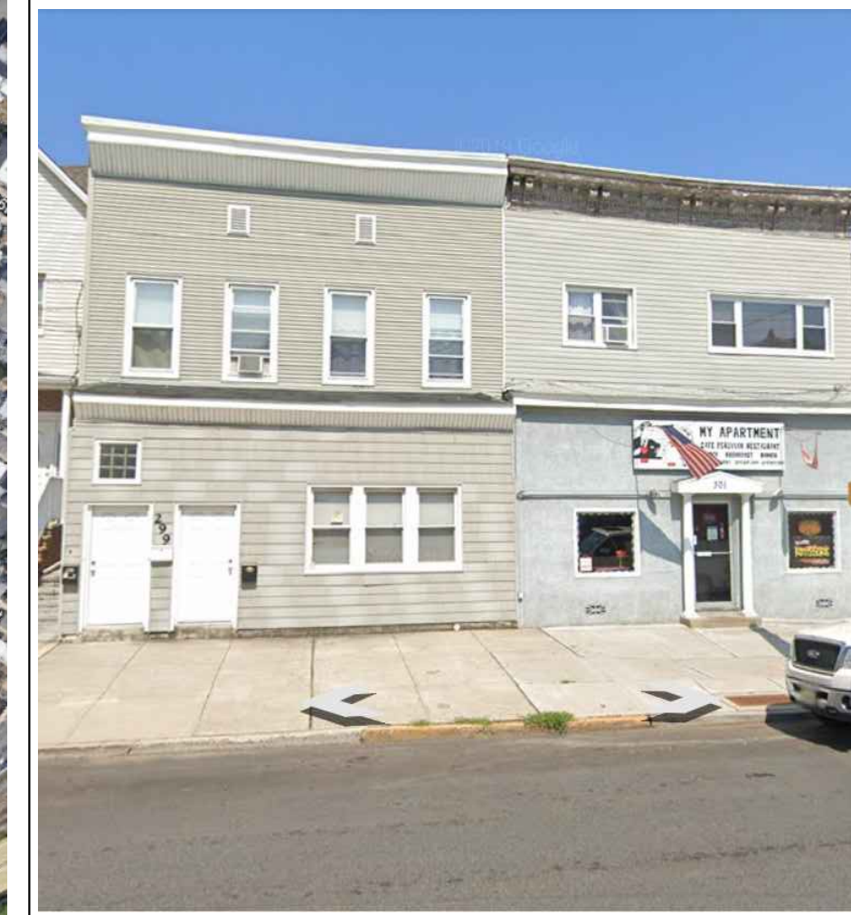
VIEW FROM AVENUE C
