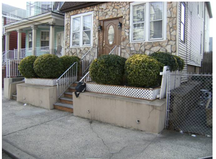
VIEW OF SIDEWALK & FRONT YARD OF WEST 17TH STREET
