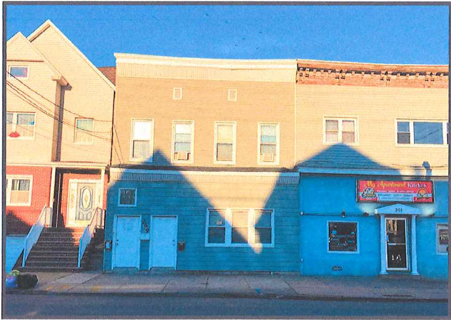
PROJECT SITE VIEWED FROM AVENUE C
